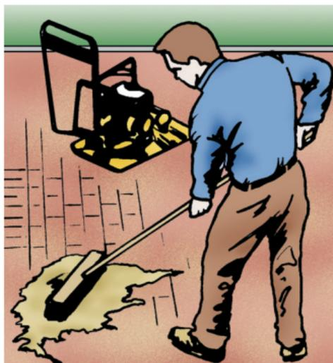
through the use of a urethane pad attached to the plate. If any of the pavers become damaged, remove them and tamp replacement pavers into place with the compactor.
