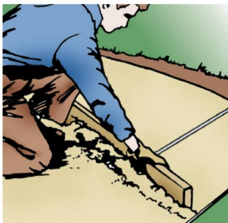
Place steel pipes on the compacted base parallel to each other about 4' to 6' apart. At several intervals, run a string line set at the height of the finished elevation across the pipes. The top of the pipes should be 1 3/4" to 2" below the line. If necessary, adjust
