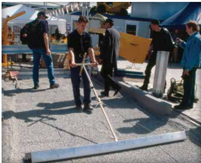
Figure 24. Manually screeding the No. 8 stone setting bed.
