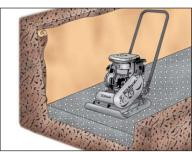
base without leaving an indentation, add the next layer of gravel. Add and compact enough gravel until the base is 6" thick with the top 6" below grade (Fig. 2). (As noted earlier, the elevation of the base will be deeper for walls over 4' high.)
