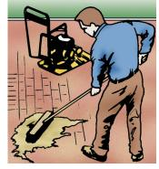
through the use of a urethane pad attached to the plate. If any of the pavers become damaged, remove them and tamp replacement pavers into place with the compactor.
