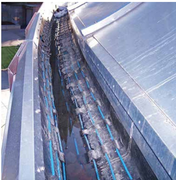
ProLine roof deicing heat cable installed in commercial gutter melt application.
