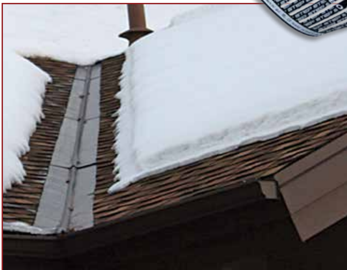
ProLine low-voltage roof heating element installed in roof valley.
