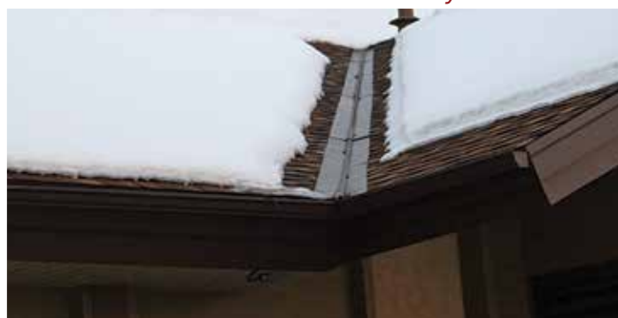
ProLine low-voltage roof deicing system heating roof valley and edge.
