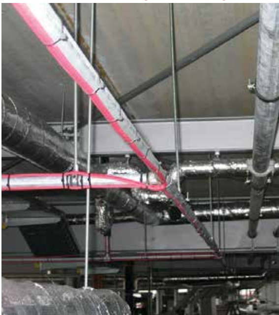
Pipe tracing system installed.
