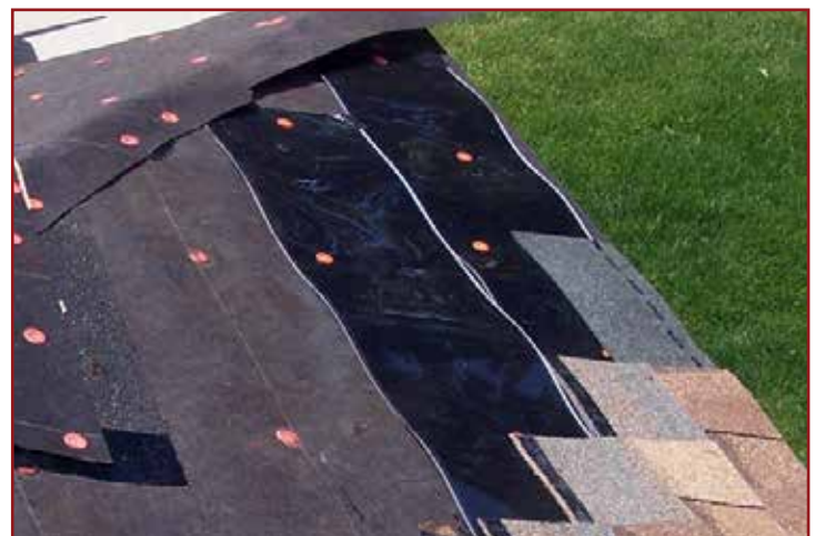
Heating element being installed under shingles.
