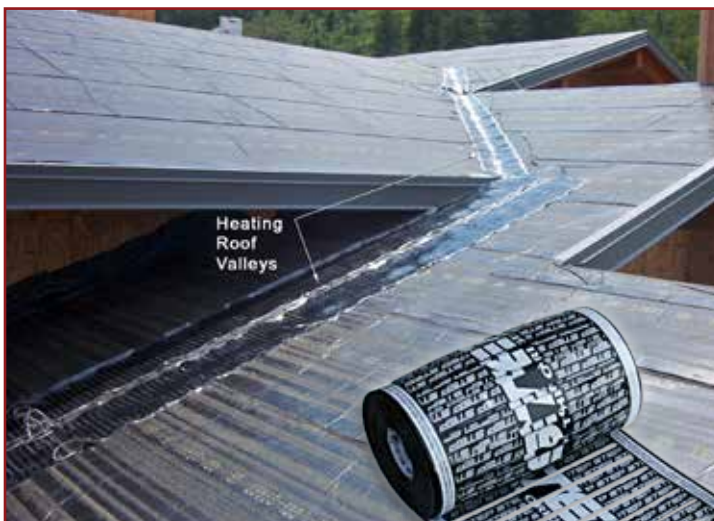
ProLine low-voltage roof heating element installed in roof valley.
