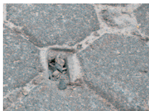
Clean aggregate is shown just below sediment deposited at the surface
